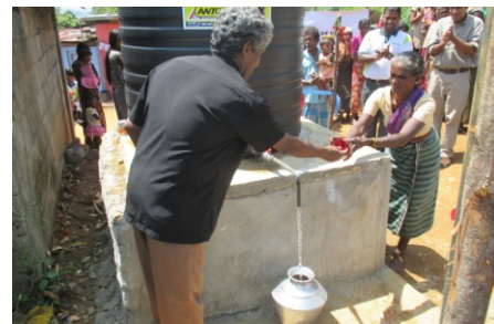
First Water from Tap
